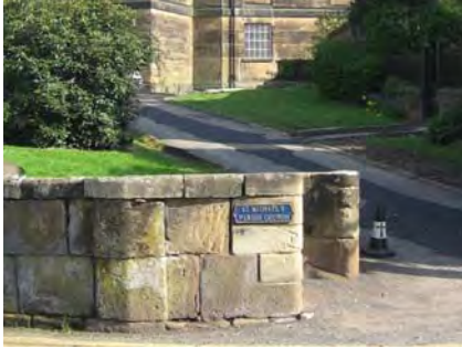
I4a Ashlar stone boundary wall
