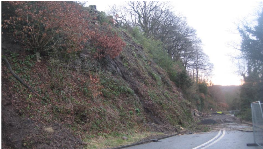
Carriageway and Footway
